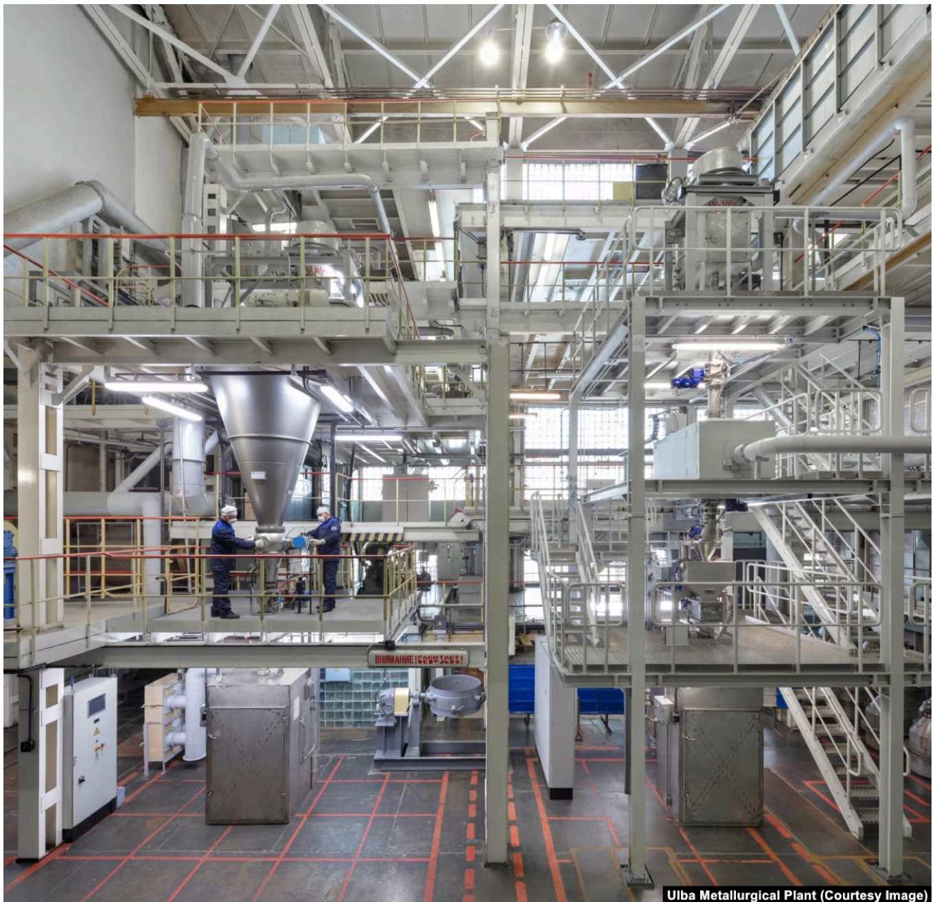
Ulba Metallurgical Plant (Courtesy Image)
